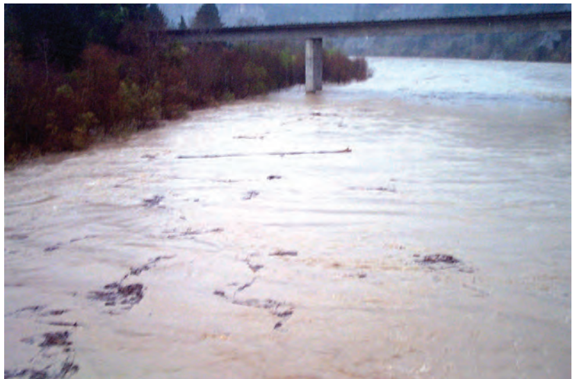
Figure A193. View of downstream bridge from streamflow-gaging station, Eel River at Scotia, California, during flow of about 200,000 cubic feet per second on February 17, 2004.
